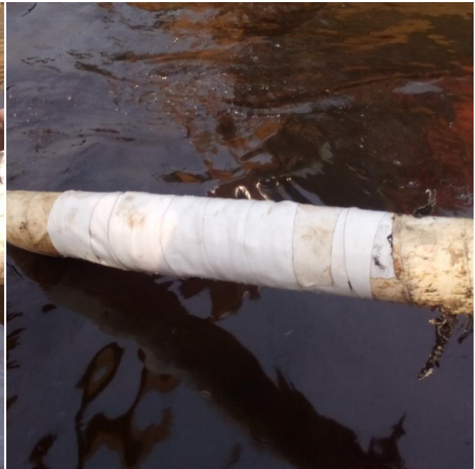
Fig F: Wrapping/Tape coating of incident facility
