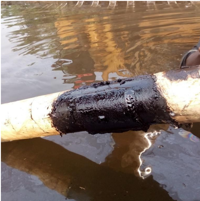
Fig E: The Leak Point Patch Welded
